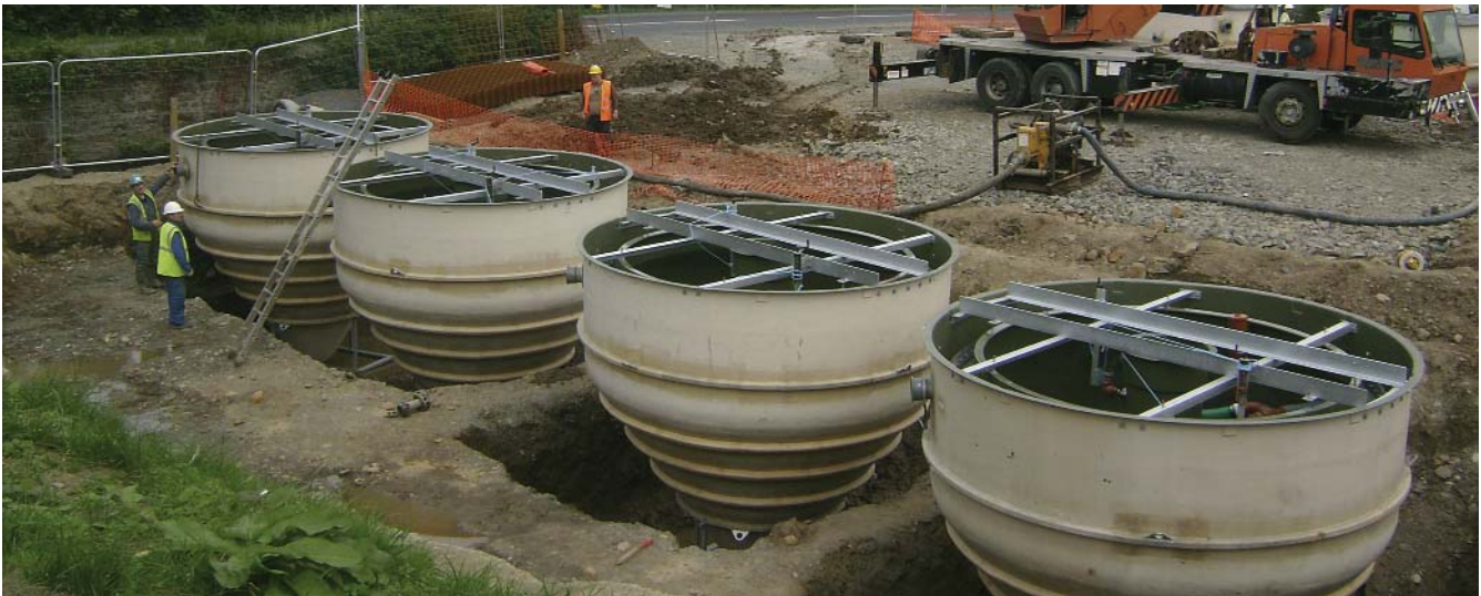
Temporary works installation
