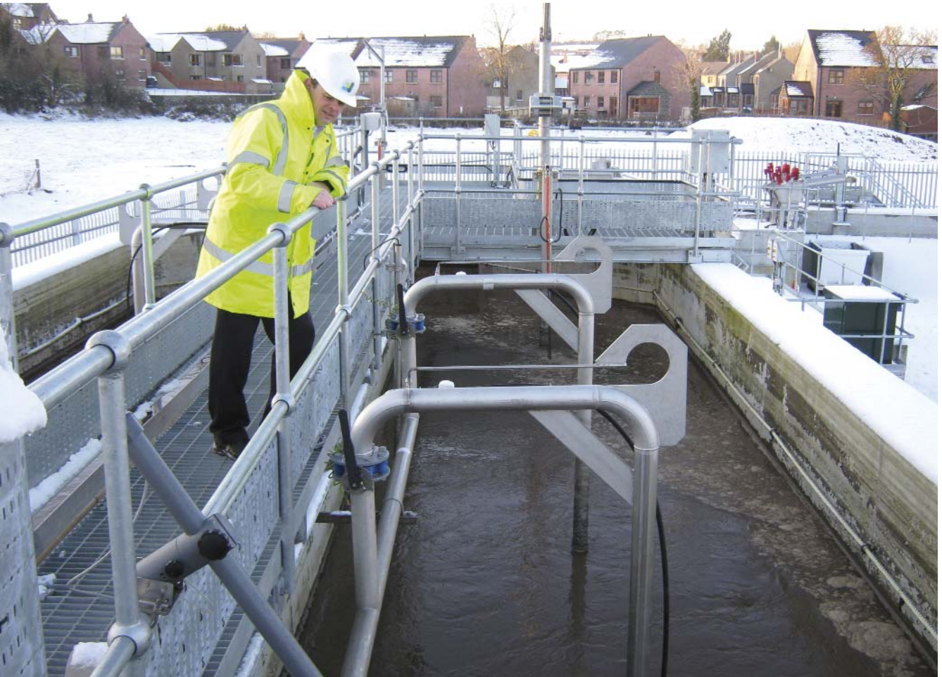
Permanent works IBA tank
