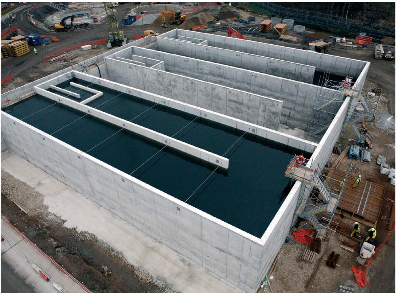
The activated sludge plant features slender walls with stainless steel tie bars
