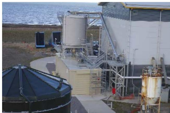
*Existing sludge building with new cake silo and loading bay. 1 of 2 new limed sludge tanks in foreground*
