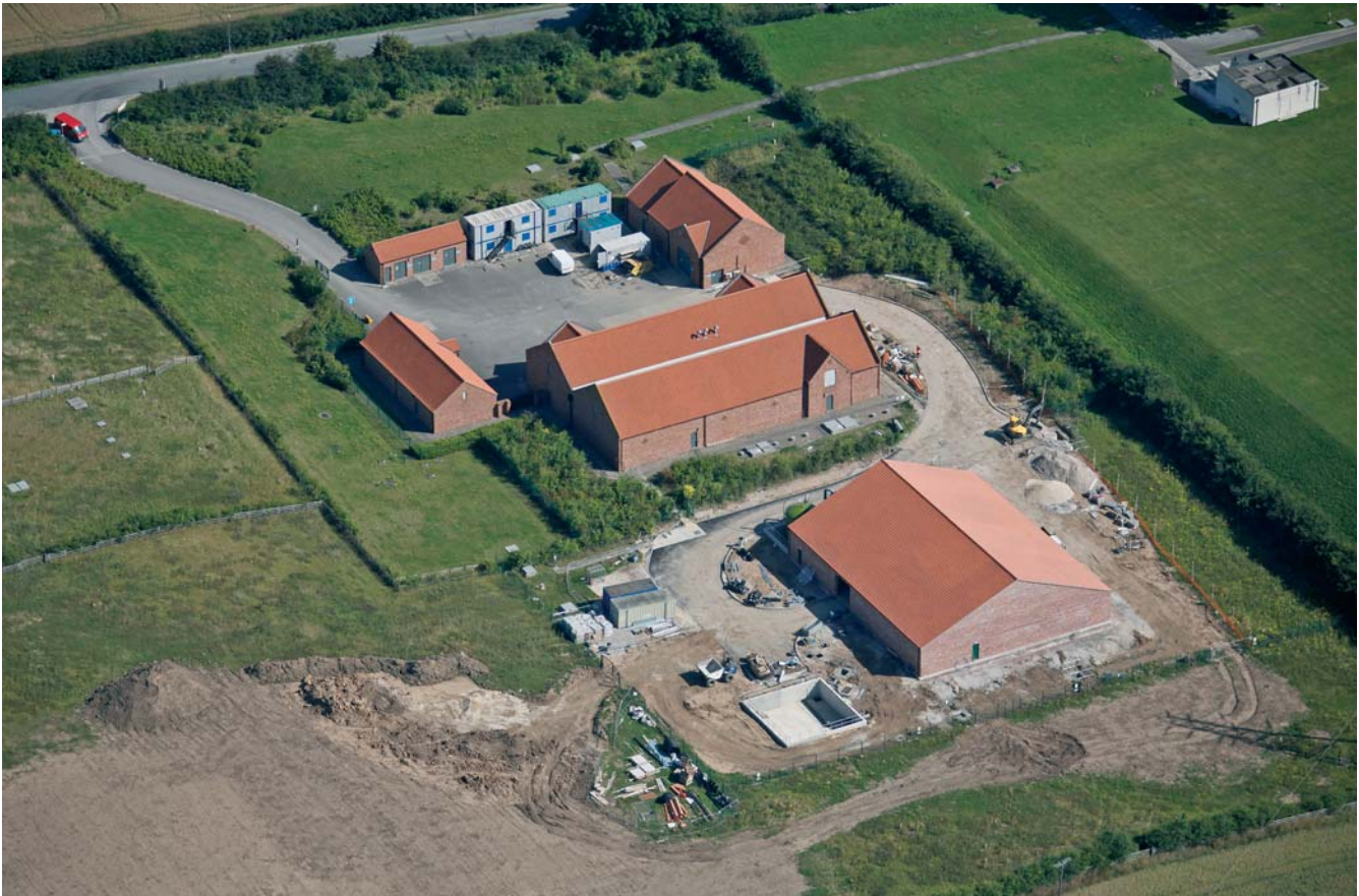
Aerial View of the Site with Civils Works Nearing Completion
