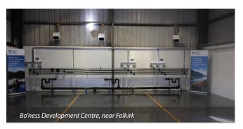
**Bo'ness Screen Testing Area**: This is a dedicated area that has been created to allow testing of new wastewater screening technologies at the inlet of the treatment works. This was achieved by installing a penstock at the inlet to create the ability to divert flows and return them prior to hitting standard screens at the treatment works.
