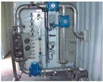
Sonix plant - stainless steel reactor under installation (courtesy Purac Ltd)
