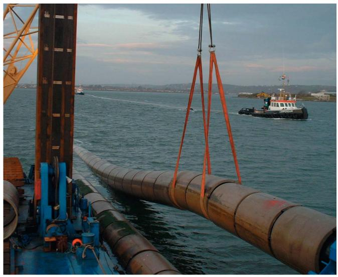
Jointing of marine pipes (courtesy E G Pettit & Company)
