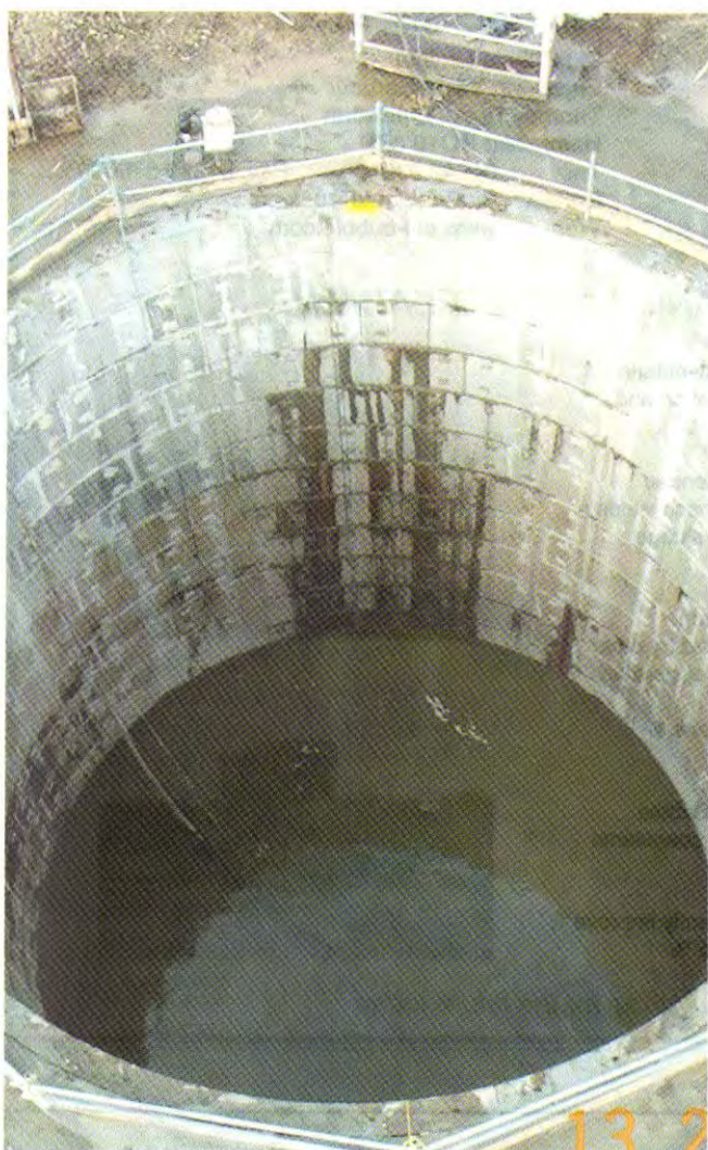
Hornsea: Sea outfall thrust bore (Courtesy Earth Tech Engineering Ltd)
