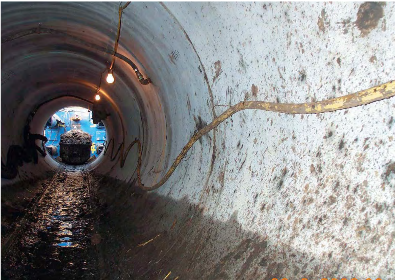
Hornsea: Sea outfall thrust bore (Courtesy Earth Tech Engineering Ltd)
