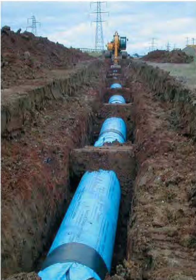
200mm pipes laid in fields (courtesy Severn Trent Water)
