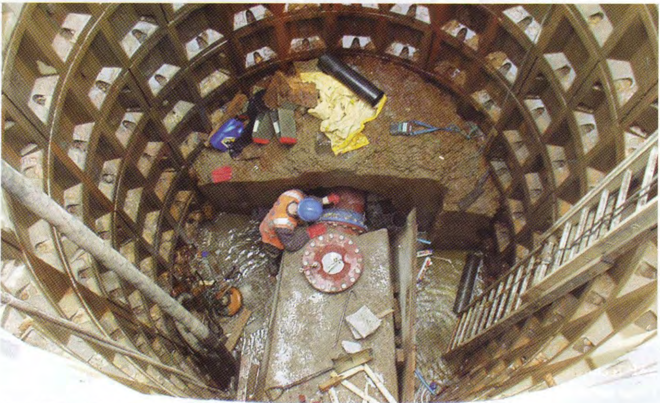
Access shaft for tunnel under railway line (courtesy E C Harris)
