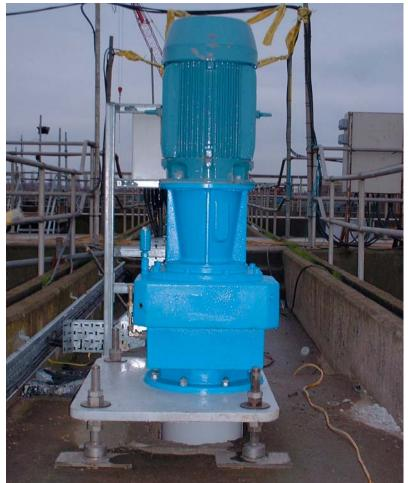
New vertical shaft aerator gear box (courtesy Thames Water Utilities Ltd)
