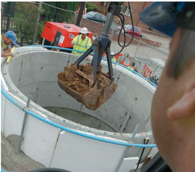
Bewdley: Small footprint 3m drive shaft (courtesy Barhale Construction).
