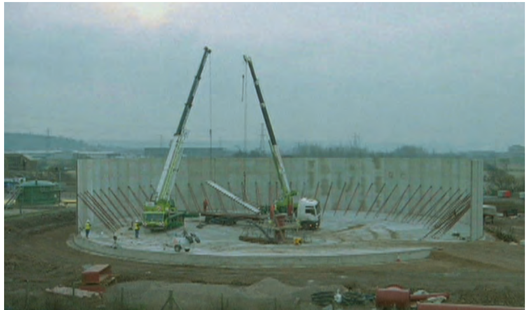
Midway through construction 10/12/02 (Time lapse photography by John Adderley, courtesy MJ Gleeson).
