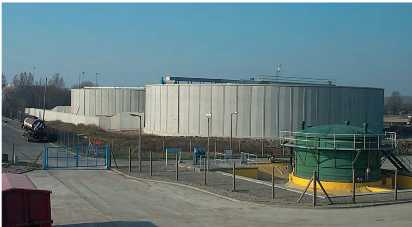
Completed tank 45m in diameter and 8m high (courtesy Wessex Water).
