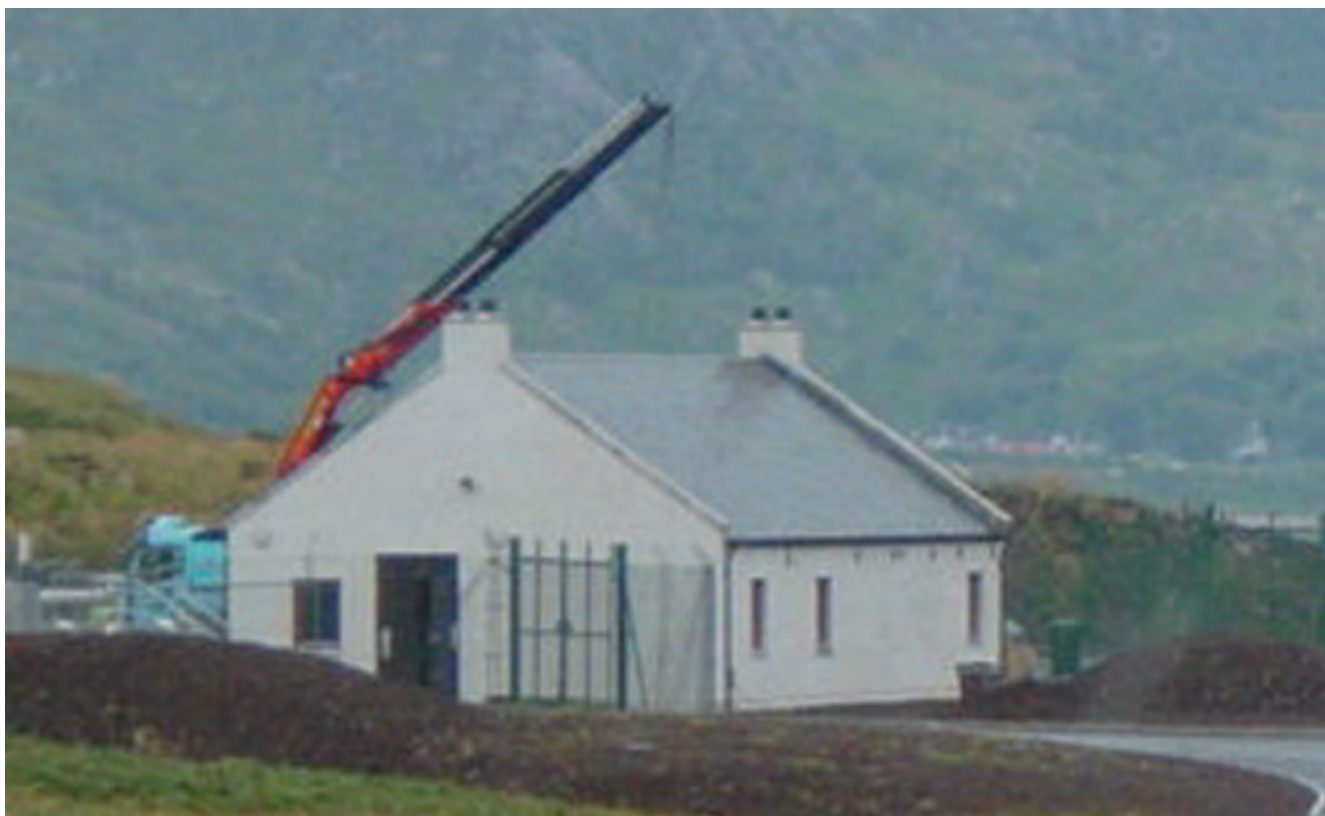
WwTW as a Crofter's cottage (courtesy Scottish Water).
