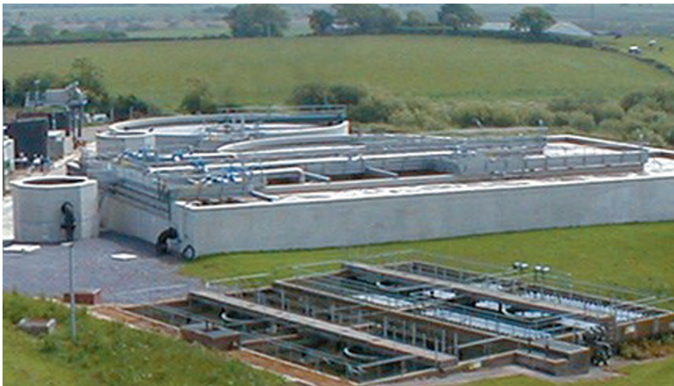
Llangefni WwTW (courtesy Meica Process Limited).
