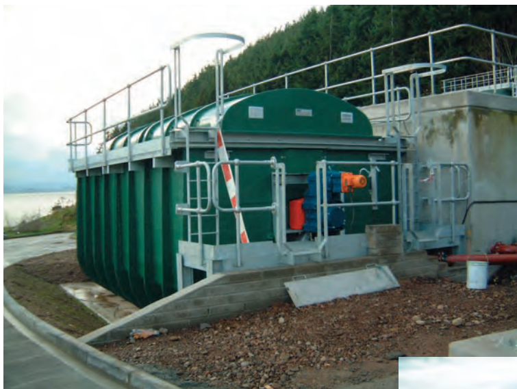
Avoch: Copa RBC - GRP tanks adjacent to original concrete tanks.
