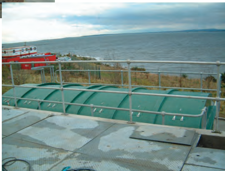
Avoch: GRP tanks & Moray Firth viewed from top of existing tanks
