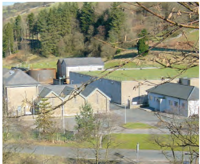
Pontsticill WTW - general view of new works (courtesy Welsh Water Alliance).
