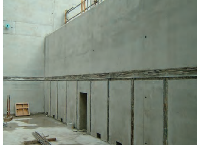
Upgrade work ongoing at Sutton Hall WTW.(courtesy Degremont)
