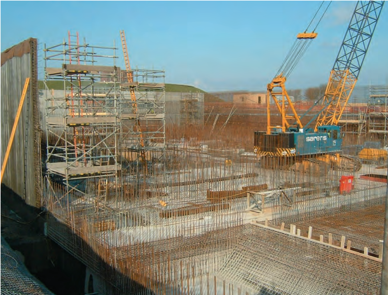
Upgrade work ongoing at Sutton Hall WTW.(courtesy Degremont)
