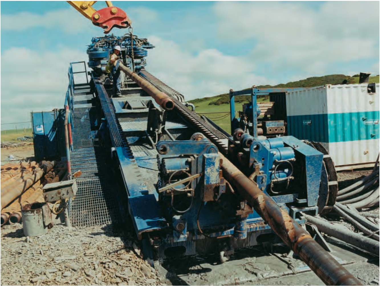
Directional drilling equipment (Copyright: Still Imaging, Chudleigh, Devon; courtesy SW Water).
