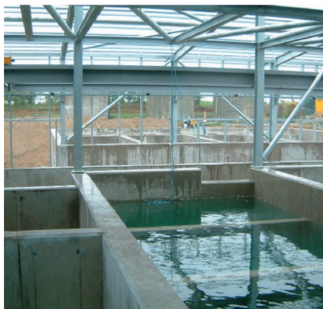
(courtesy Earth Tech Engineering Ltd)
