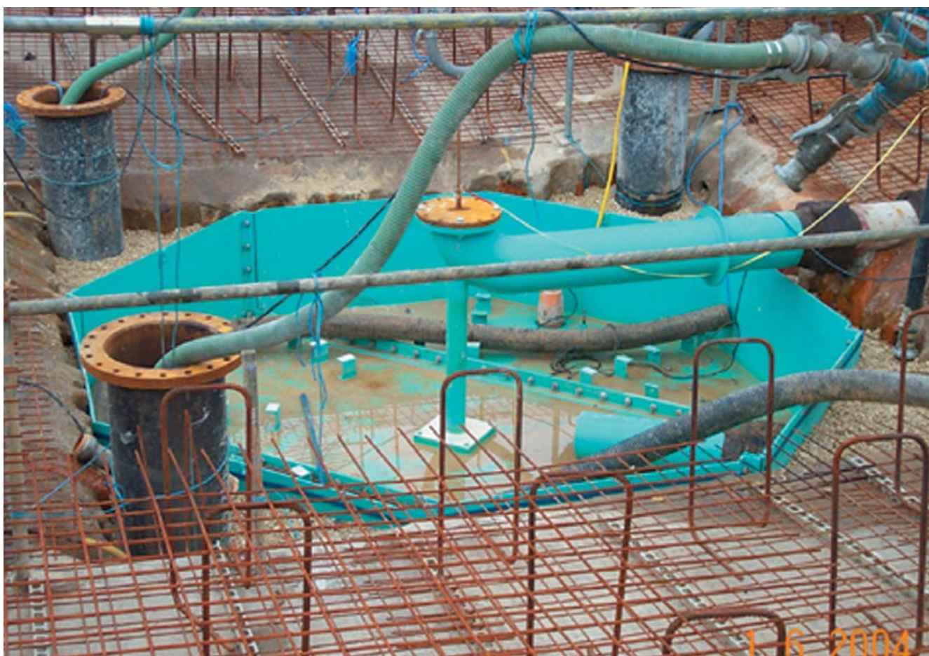
Removing groundwater for construction of final settlement tanks
