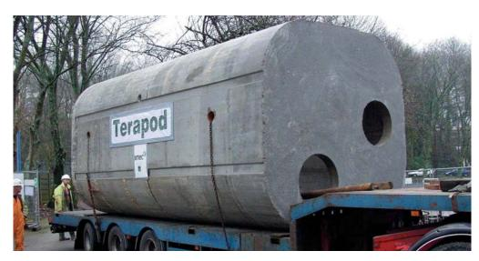
The 'Terapod' An alternative method for constructing the concrete CSO chamber. It was pre-cast off site and delivered 'on the back of a lorry'. Reducing 'curing' time, hire of ground support systems, disruption to roads network and the community.
