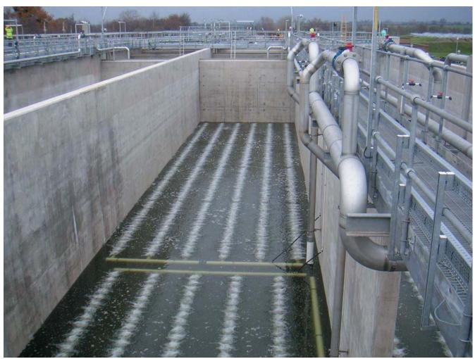
Hartshill: ASP2 aeration lanes, fitted with diffuser grids of varying densities.
