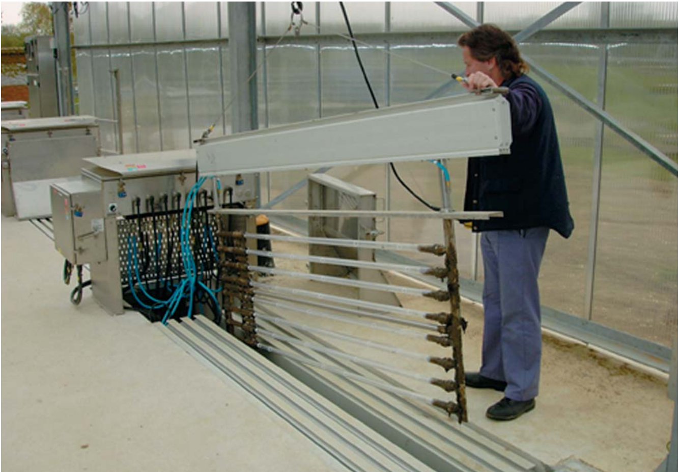
Installing tertiary UV disinfection at Wessex STWs
