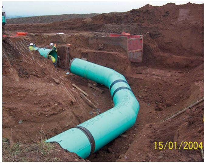
Melbourne WTW: Installation of welded steel pipe
