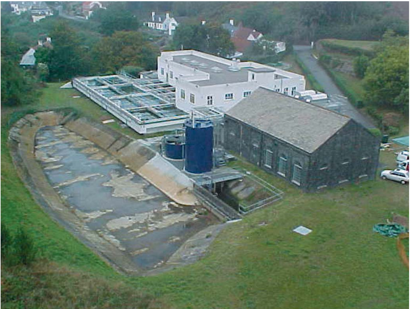
St. Saviours Water Treatment Works, Guernsey
