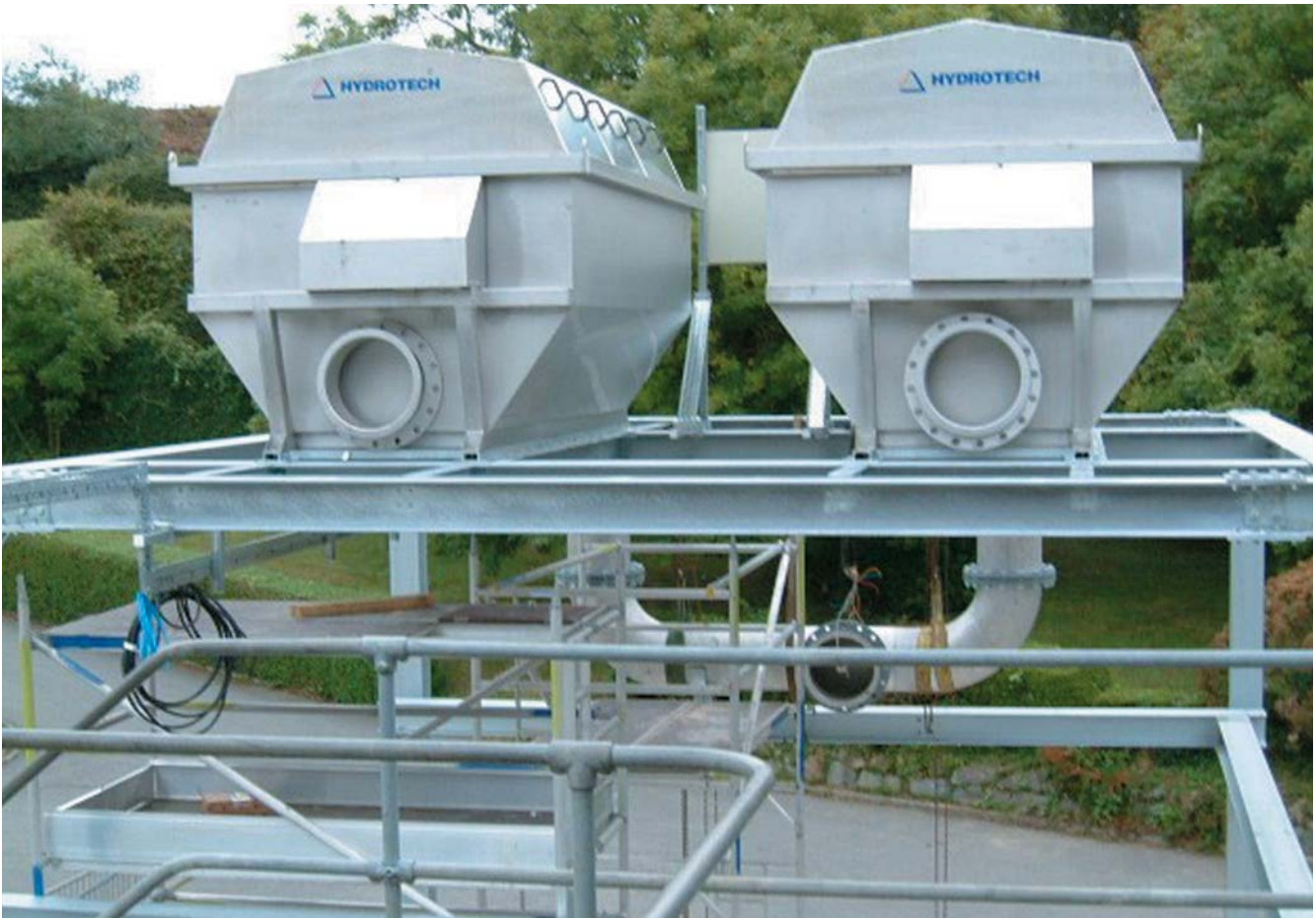
Inlet micro-strainers at St. Saviours WTW
