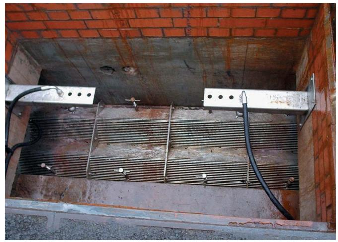
Stoke-on-Trent: Fixed screen with cleaning equipment
