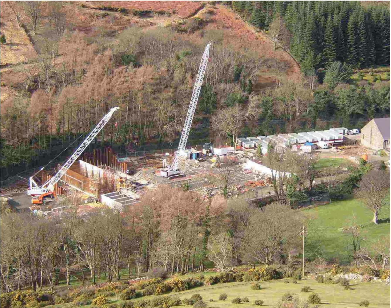
Sulby, Water Treatment Works under construction
