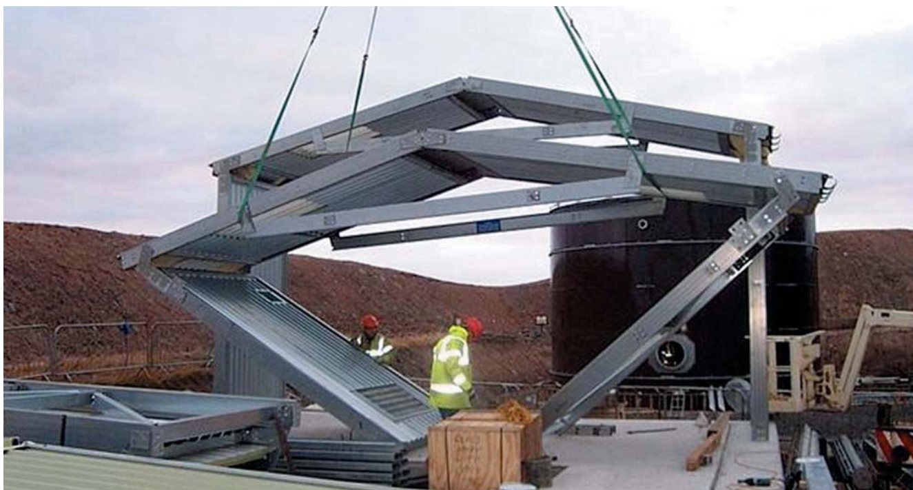
Erection of the Kitpac sectional building
