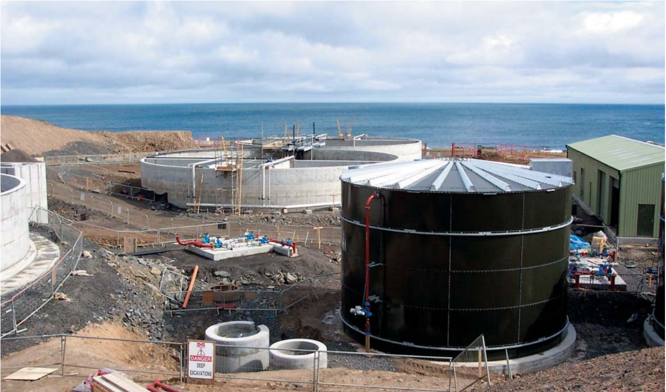
Wick, Caithness, Scotland WwTW under construction
