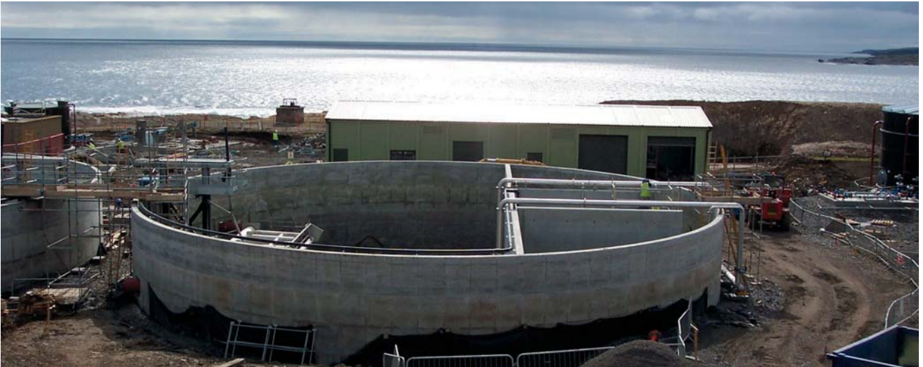
Wick WwTW facing South over CASS
