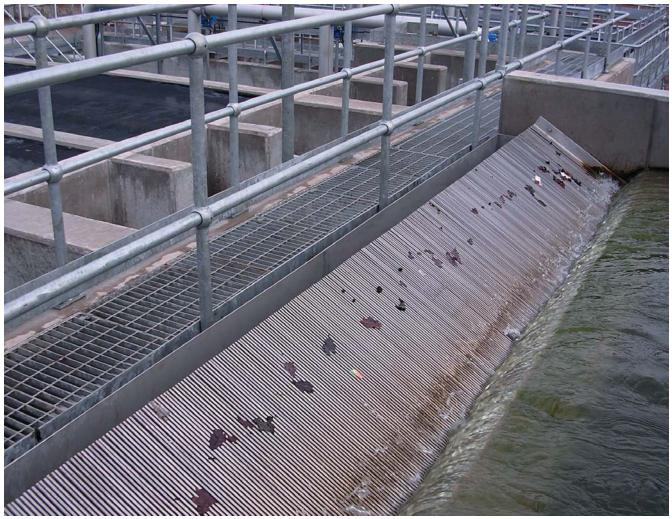
Worksop STW: Manual screen on inlet to protect proprietary T blocks
