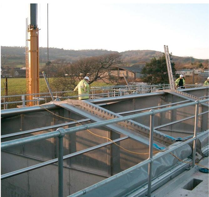
Charmouth STW: Rollback covers fitted to SBR tanks
