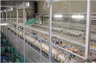
View of top of CMF5 units showing the filtrate and air headers courtesy: Black & Veatch Limited
