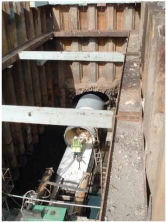
Shield and first pipe prior to jacking within the sewer
