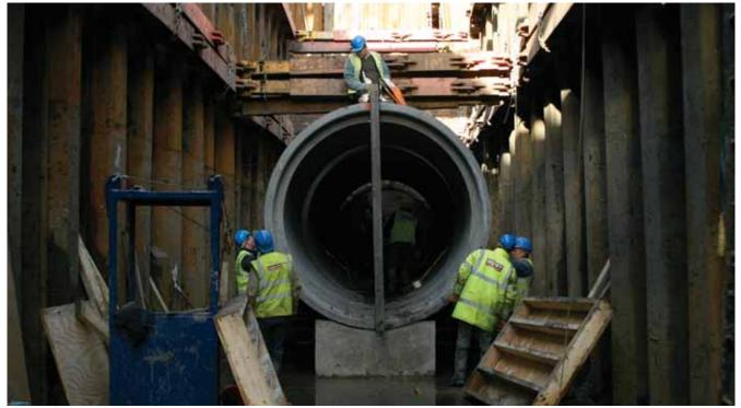
Knostrop Sewer: Placing of concrete pipes - note man standing upright inside pipe
