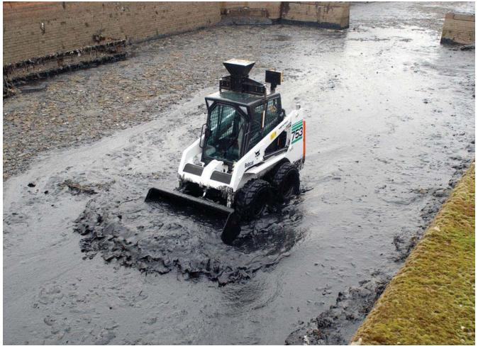
Knostrop STW: A remote controlled 'Bobcat 753 which can clear sludge up to 3 m deep from storm tanks
