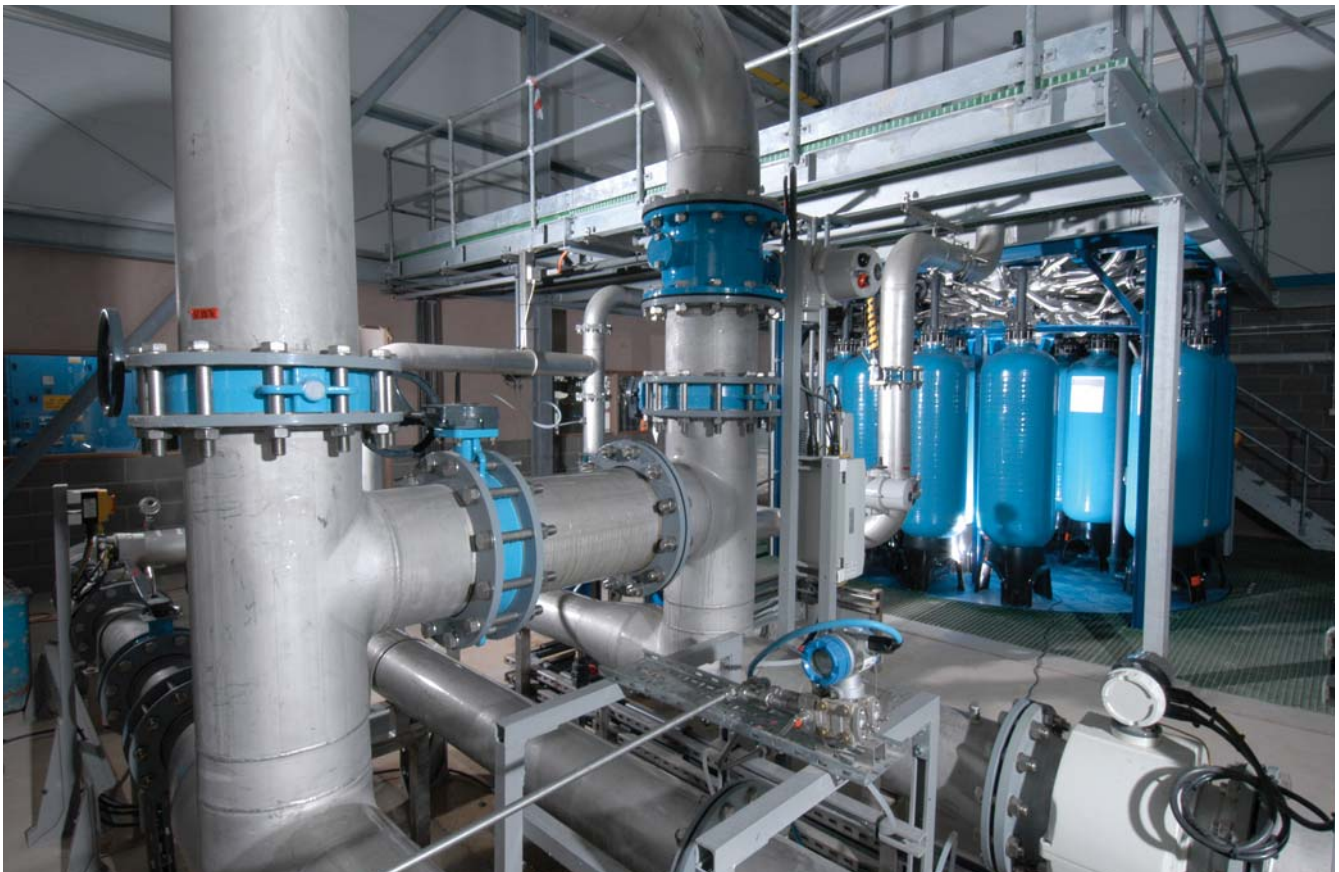
Lane End: View of ISEP plant with blending by-pass in foreground
