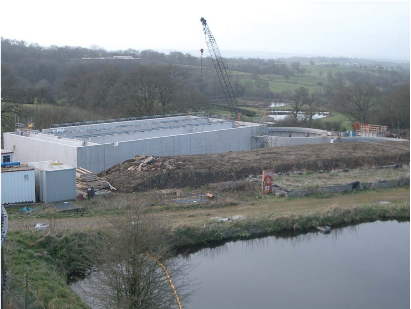
Shaftesbury STW: General view of construction works
