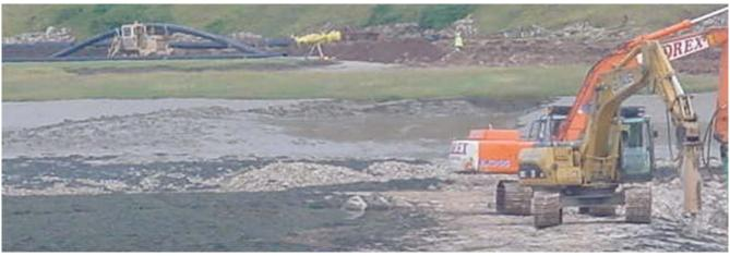
Construction of Aust outfall. Trencher in background working on salt marshes
