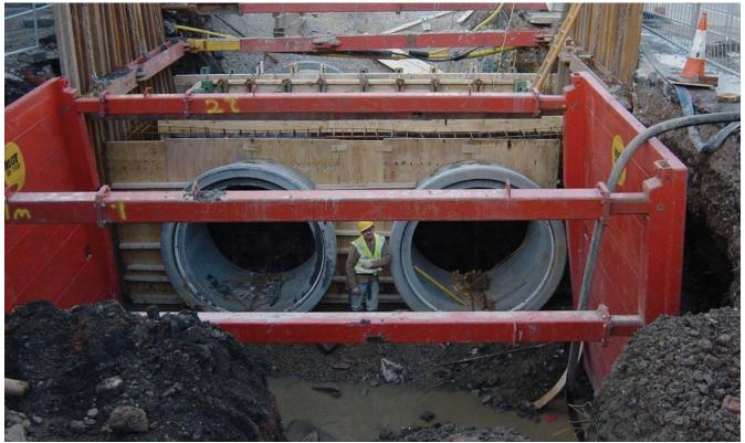
Totley Brook Road: Twin 1800mm pipes being installed in urban area
