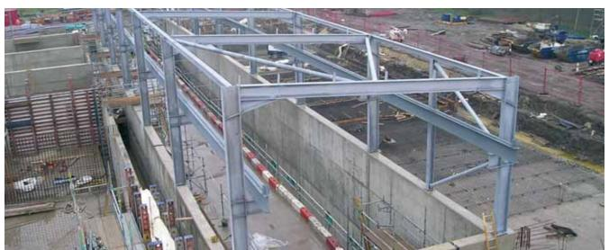
Loftsome Bridge: Steelwork erection to central gallery of DAF units
