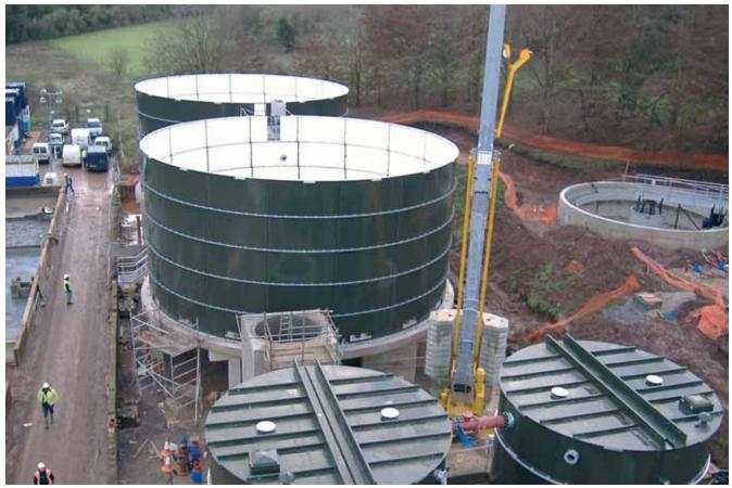
Paulton STW:Sludge holding tanks (foreground); trickling filters/primary tank (background)
