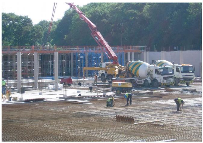
Northern Startegic Support Scheme - reservoir under constrcution showing column casting rig
