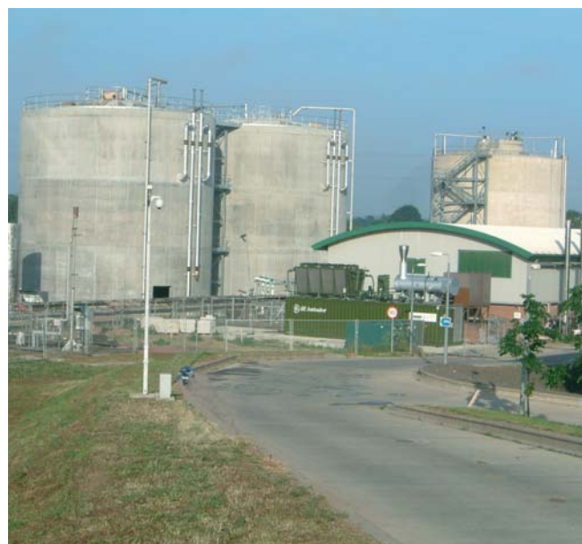
View of Digesters 7,8 & 9, Boiler House and CHP Plant courtesy Nomenca Ltd
