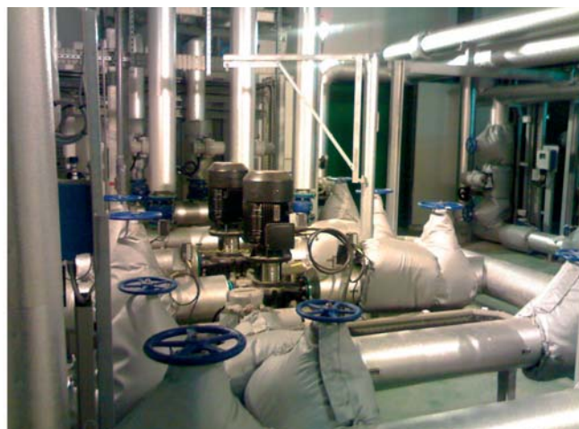
3D Model View (left) of Digester Hot Water System (courtesy of Nomenca Ltd) and view of 'As Built' (right) Digester Hot Water System (courtesy of Severn Trent Water Ltd)
