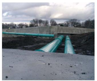
The new rising main (right) feeding the activated sludge plant and the return main (left)
