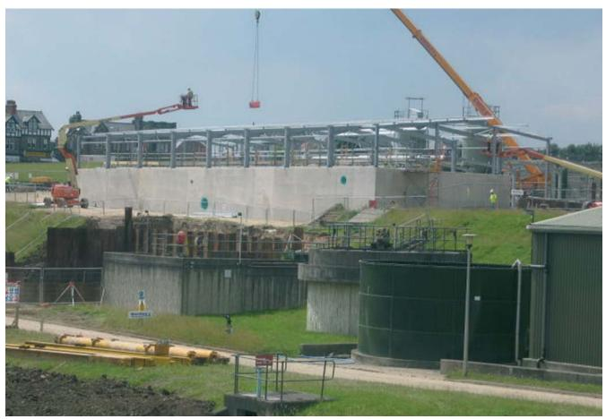
Erection of steelwork frame to newly constructed rapid gravity filter substructure
