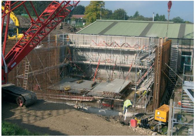
Harlow Hill WTW; Construction of clarification unit under the regime of continually operating live treatment process
