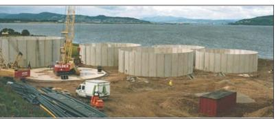
Aqua-Tanks being installed at Inverness – the concrete panels are held together by means of a high-yield steel tendon system
