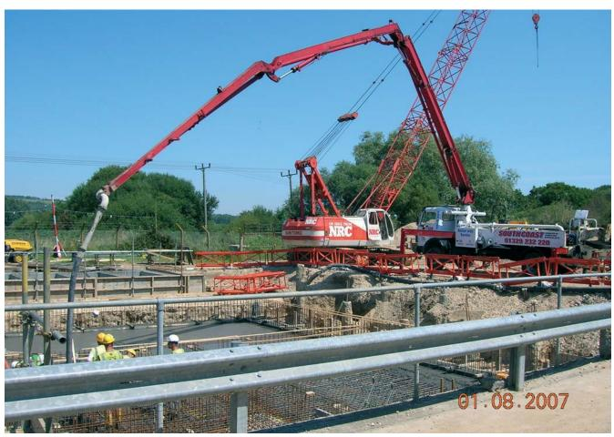
concrete being poured into the base of the new wash water tank
