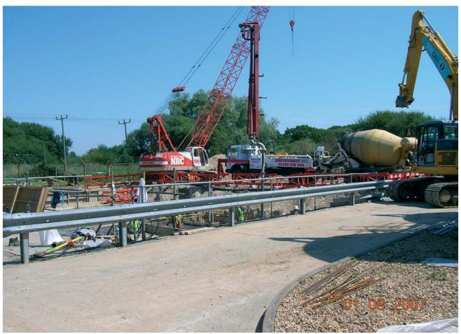
concrete being poured into the base of the new wash water tank
