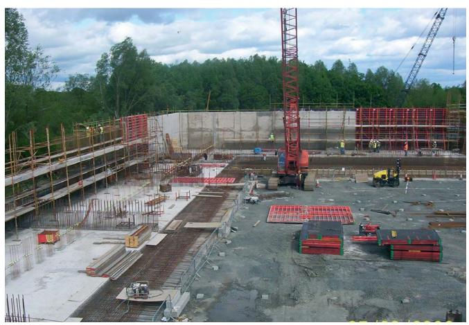
Phased construction progress of the SBR structure to maintain access for concrete pours
