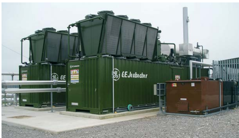
Blackburn WwTW CHP installation
