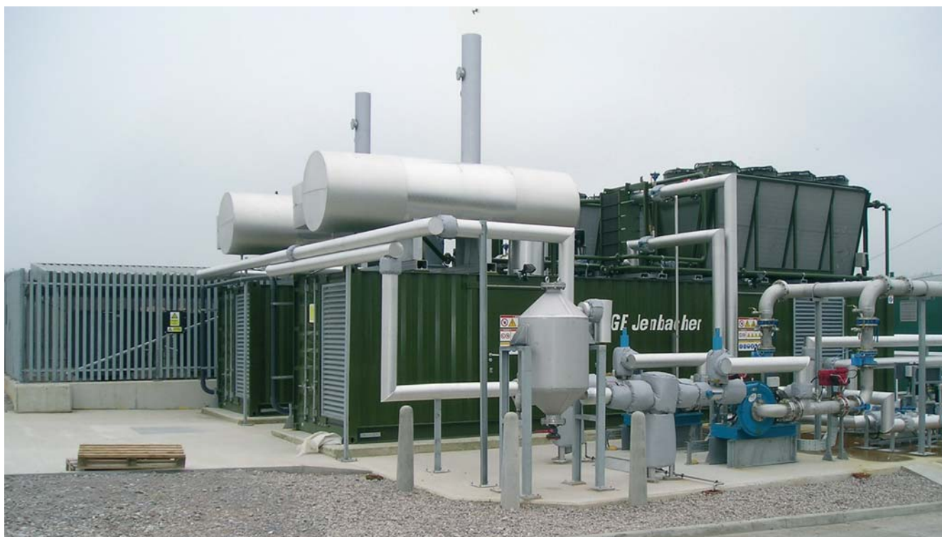
Blackburn WwTW CHP Installation
