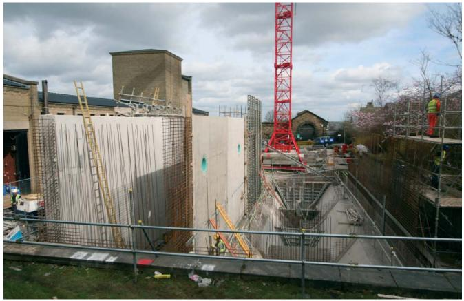
Albert WTW: Ongoing construction of the contactor and resin separation tanks
