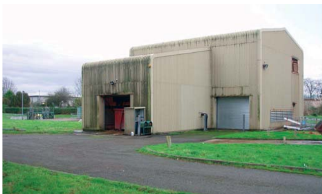
The old screens and screenings were housed in this building (left) & demolition (right)
